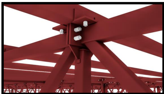
Pic.4. Cross truss connection unit
